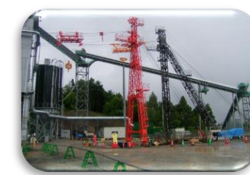
Cable cranes for transport equipment for renovation of hydraulic power generation
